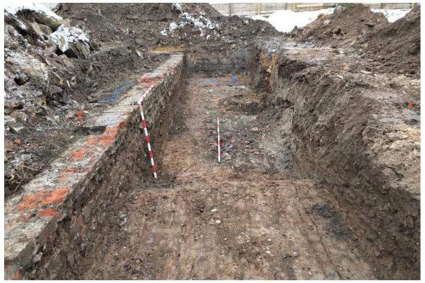
Plate 5: Showing soil retention wall (104). Well structure visible in background. Looking east, one and two-metre scales.
